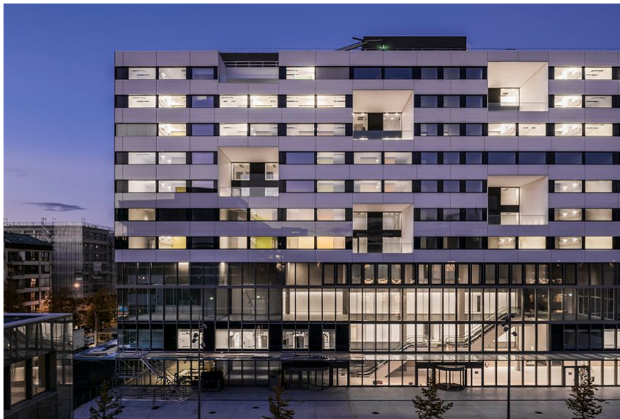
University Hospitals of Geneva - Gustave Julliard hospital building
